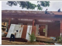
Boarding house in Turn secondary before remodelling
