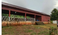
Dinning building in Turn secondary school before remodelling
