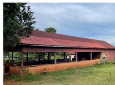
Dinning building in Ochum before remodelling
